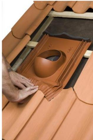
**ENG:** Make sure there are no sharp edges in the tile under the seal. If the tile is high, you should bevel the end of the tile which comes under the corrugated rubber. This makes the installation look nicer. Remove the protective film from the bottom of the corrugated rubber, and hammer the corrugated rubber tightly straight against the roof tile from the entire width of the seal.
