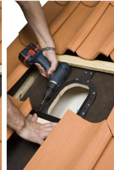
**ENG:** Attach the bracket to the side of the lowermost batten with two long screws. Check that the sideways location is correct.
