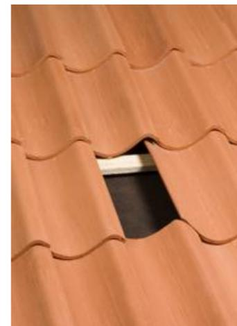
**ENG:** Remove one tile to which you will install a Universal tile pass-through. Make sure there is not a roof truss at that spot.
