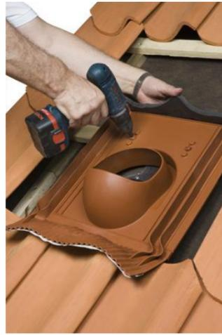
**ENG:** Mount the top part of the pass-through onto the batten with two short screws. Choose an appropriate seal of the three seal alternatives for the top edge of the pass-through. Remove the protective film of the tape from the pass-through, and mount the seal onto it. Make sure that it is in the correct location sideways.
