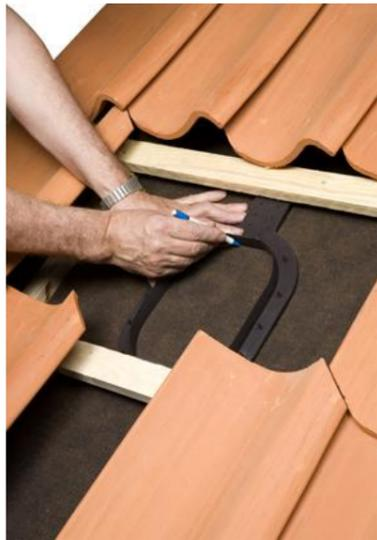
**ENG:** Mark a hole in the underlay by using the underlay seal. The seal must be attached to the lower batten.
