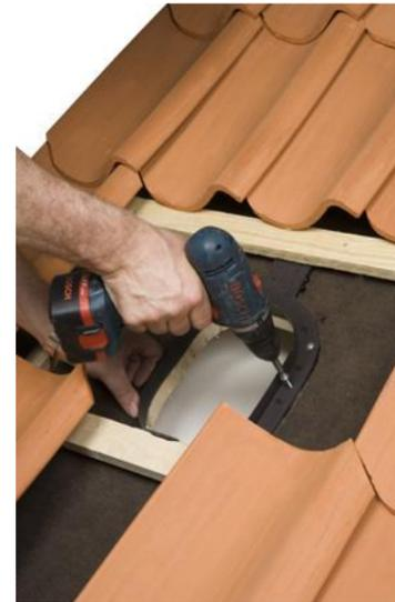
**ENG:** Mount the underlay seal onto the wood through the underlay with screws. If the underlay is made of plastic and there is no wood under it, put the underlay seal under the plastic, so that the spikes go through the plastic. Press the plastic tightly against the silicone and screw down the screws in the upper and lower battens.
